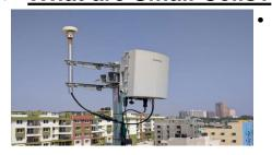
Small cells are low-powered radio access nodes or base stations that have coverage range from a few metres up to a few hundred metres.
